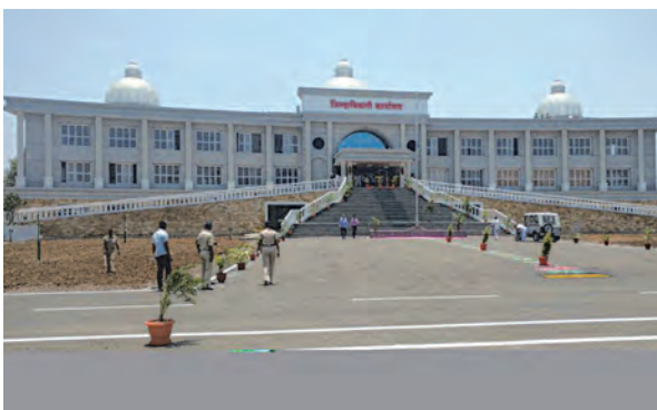
District Collector Office, Sangli
