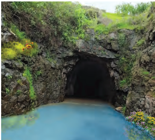
Devsane (Manjarpada) Project : Tunnel
