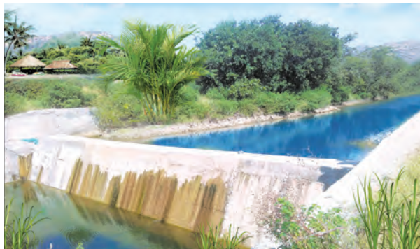
Nala Bunding –cement nala bunding
