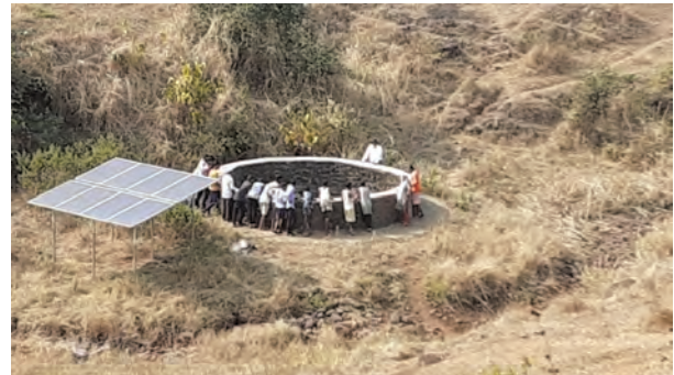
Construction of well through public participation
